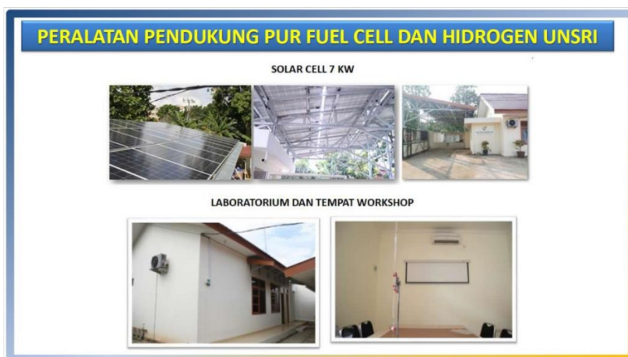
Figure 1 Example of buildings powered by solar panels.
